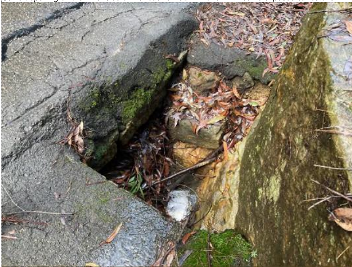
Culvert opening on the inner side of the road with some exposed sandstone.
