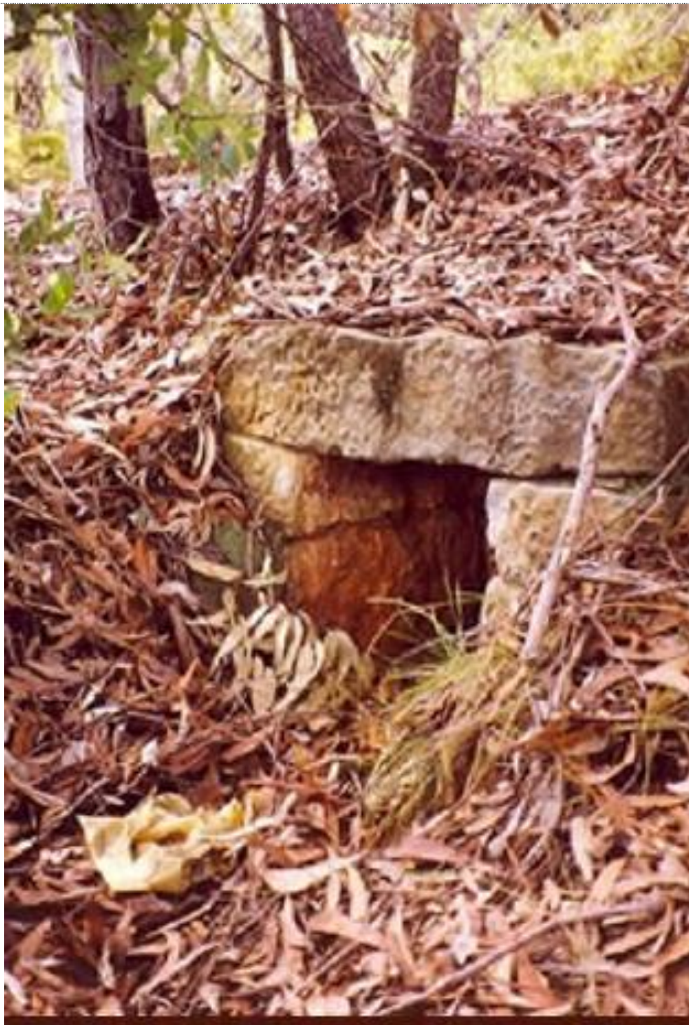
Culvert opening on the outer face of the road, located behind the fence on the roadway.
