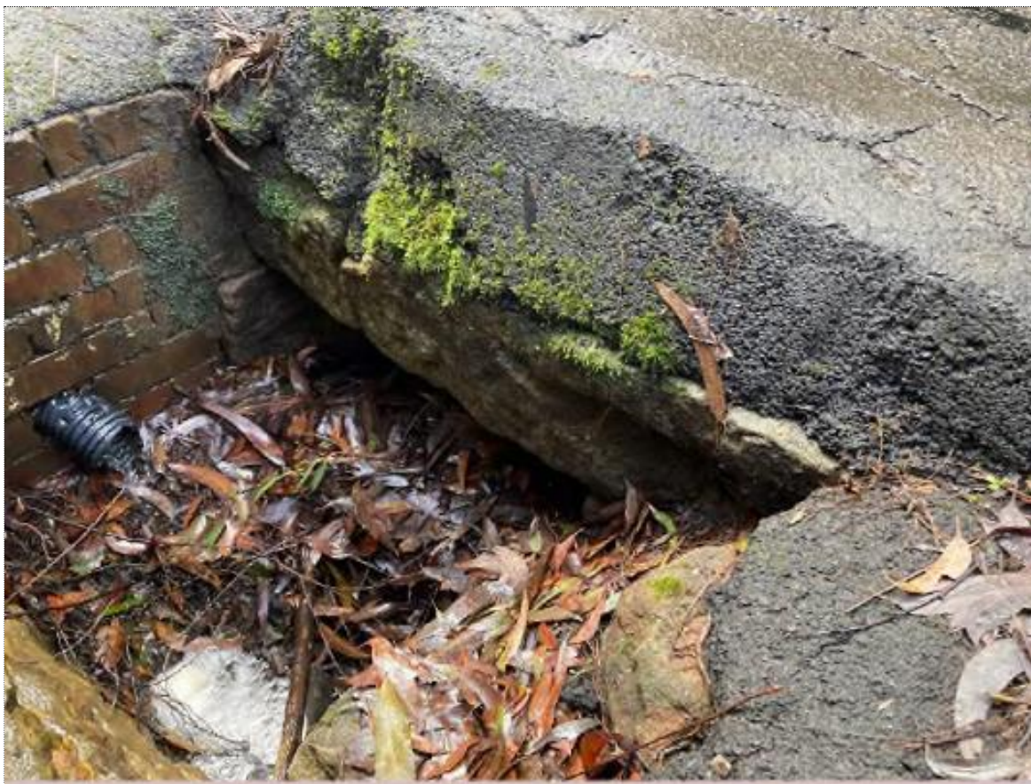
Culvert opening on the inner side of the road relined with brick with some exposed sandstone.
